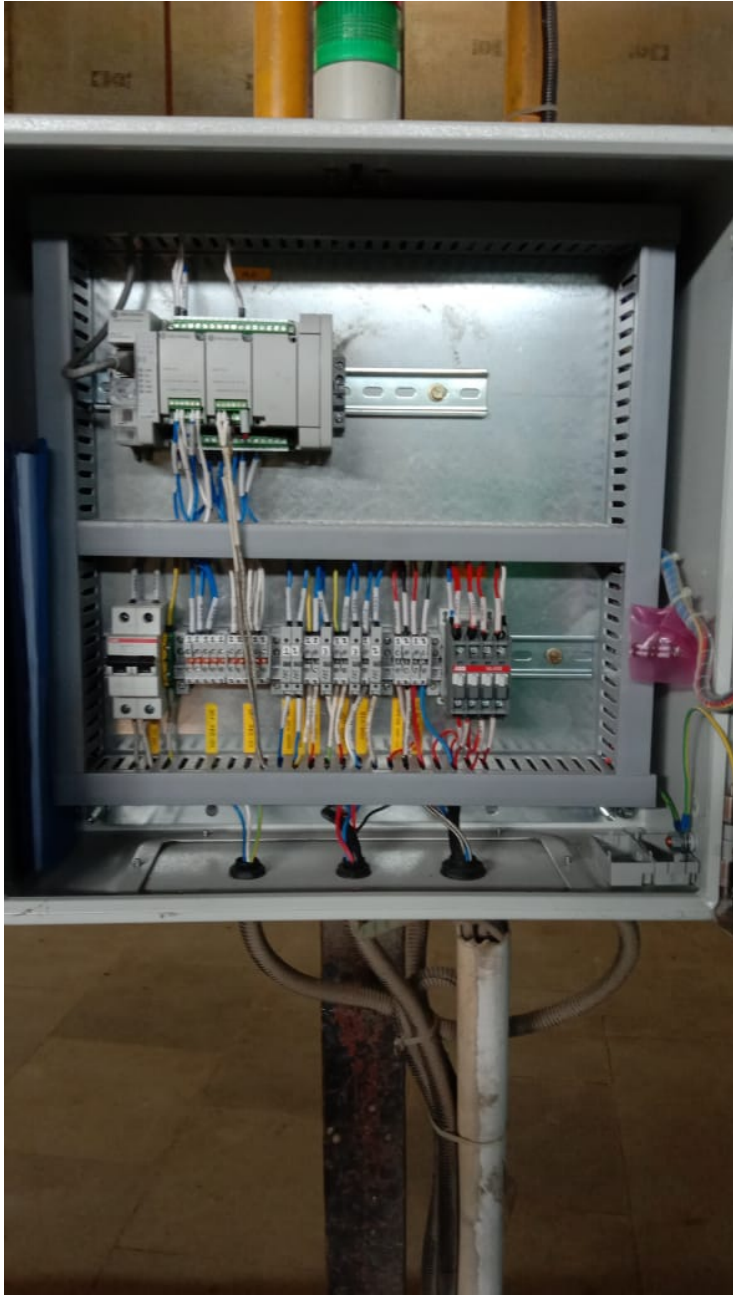
Electronic( Plc) Controle Pannel Fitted With Kit. Sensors exhaust temp, Map, Mat & engine vibration (Vib.) fitted on engine as required
